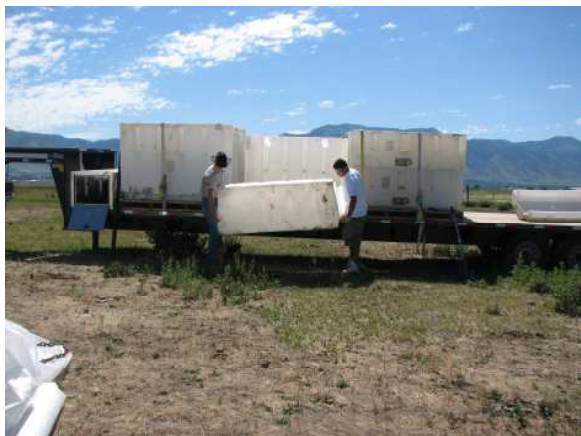
(Step 1) Lift the 110 pound Muscle Wall Avoid Dropping
