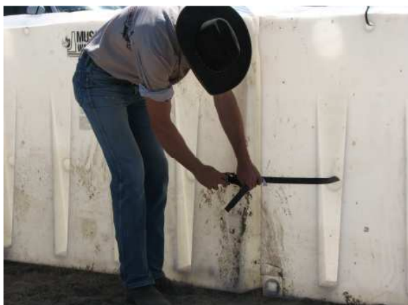
(Step 3) Ratchet strap around each connection
