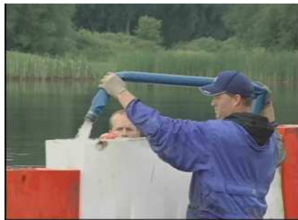
(step 9) Fill each Wall completely with water
