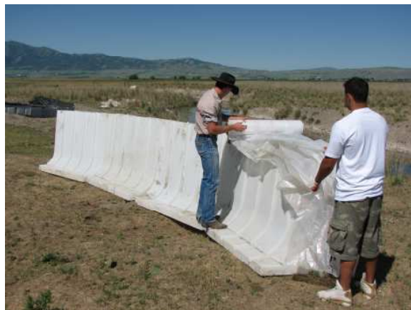
(Step 4) Roll out the poly-string plastic Plastic-Sheet must be used
