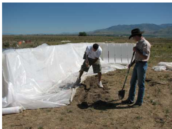
(Step 6) Dig a six inch deep trench Do NOT pull plastic sheeting tight
