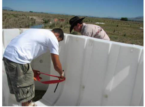
(Step 8 A) Loop red-strap around rebar strap
