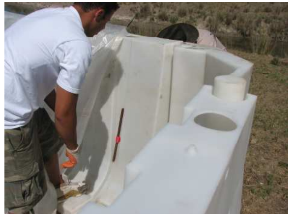
(Step 8 B) Tighten red-strap evenly
