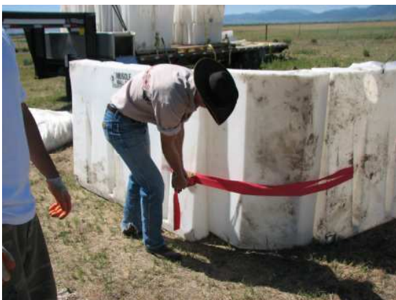
(Step 8) If using a corner wall, use red-straps
