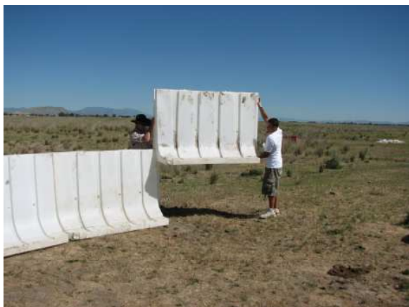
(Step 2) Slide wall onto opposing connector
