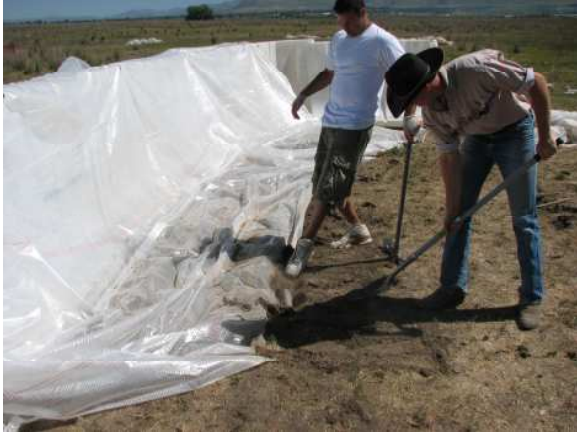
(Step 7) Bury the edge of plastic to create seal
