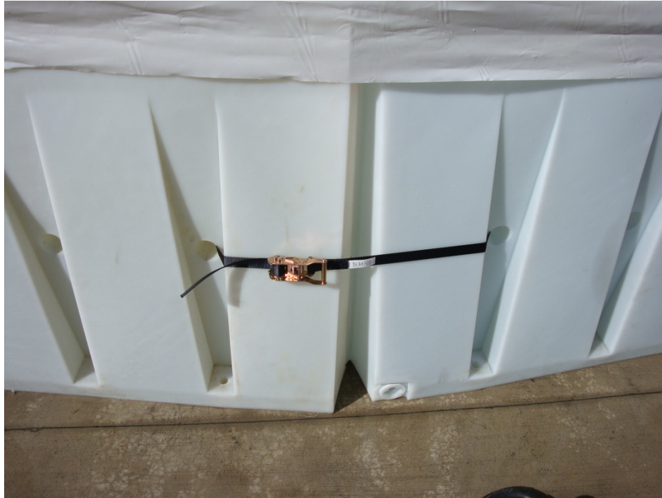
Figure 5. Strap used to secure walls together.
